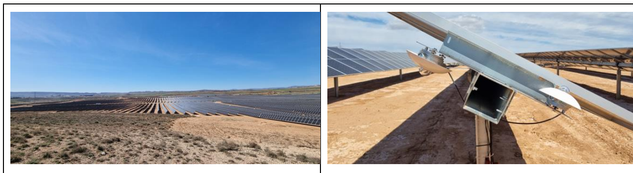
Figure 5.1: Pitarco PV plant
