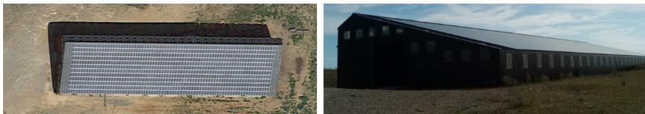
Figure 5.2: SANT PV Plant aerial and on-site view
